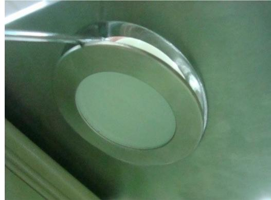
5. Pull the illuminant carefully out of the hole and disconnect the energy supply wire.
